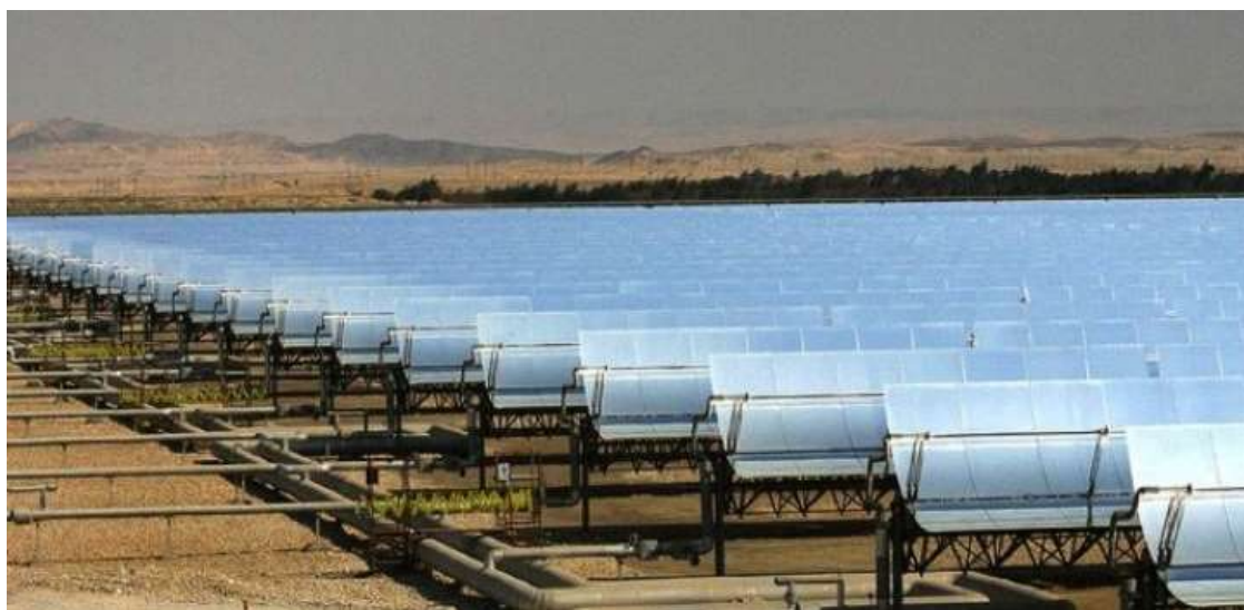
Figure 4: Parabolic Trough Technology ( www.e-education.psu.edu )
