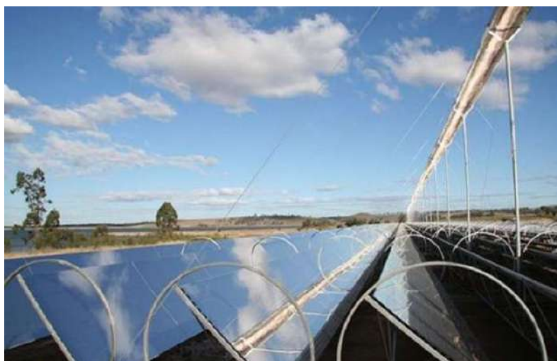
Figure 7: Linear Fresnel Reflector Technology ( social.csptoday.com )
