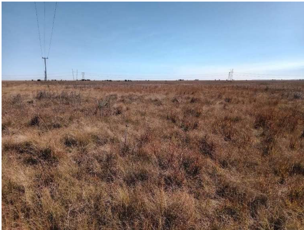
Figure 18: View over the northern section of the longer powerline route option (Alternative 2)
