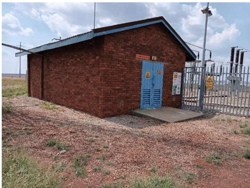
Figure 38: Building at Eskom substation
