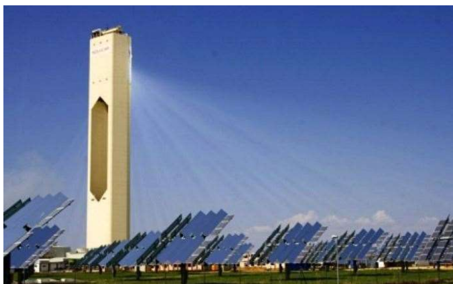
Figure 5: Power Tower Technology (Planta Solar 10, Spain)
