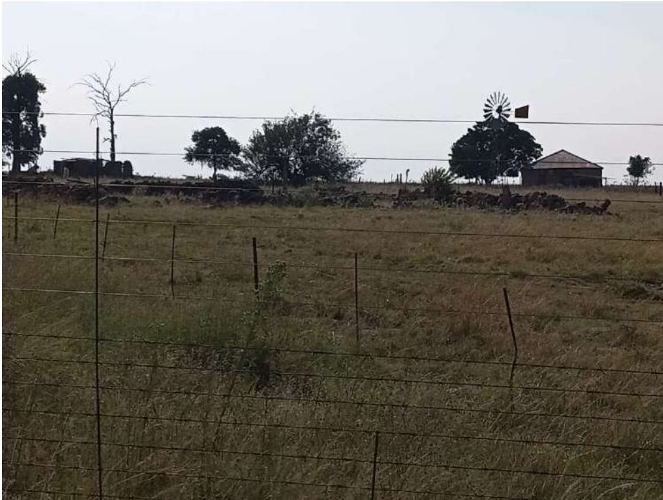
Figure 26: View of the three historical structures located at Groot 01. It was not possible to obtain a closer view due to fence and no gate.
