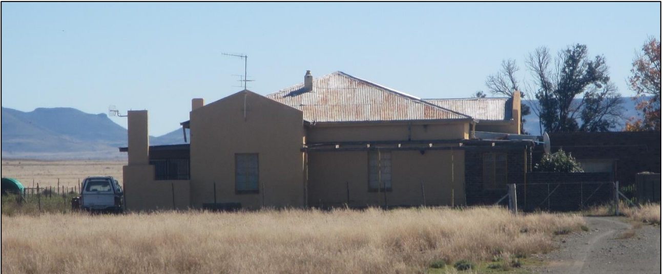
Figure 36: Farmhouse at waypoint 932.
