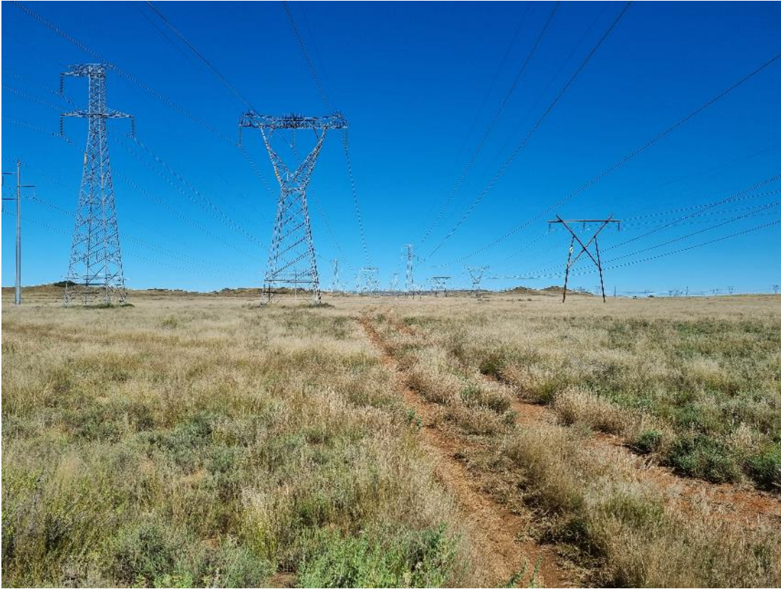
Figure 9: Existing HV powerlines within the PAOI
