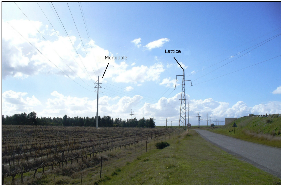
Figure 4: Typical 132 kV power line structures
