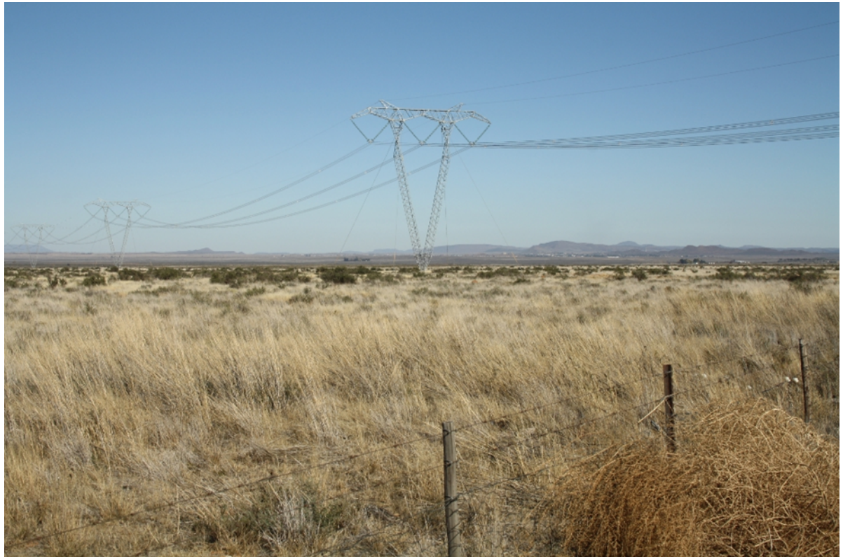
Figure 5: Powerline infrastructure within the region (note the shrubland vegetation)
