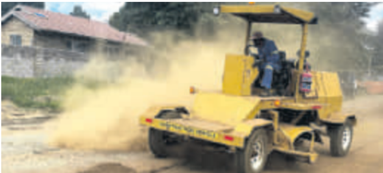
Municipal workers during the construction of Horster Road.
