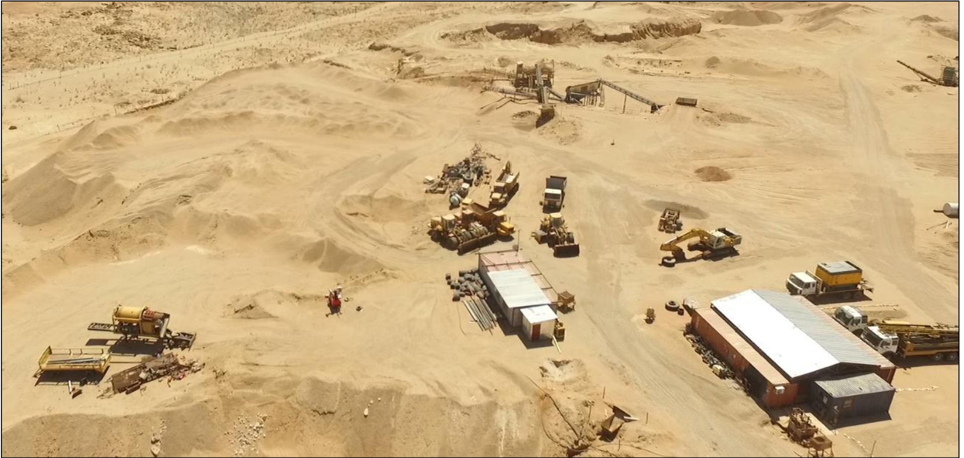
Figure 9: Workshop 1 with parking and laydown area
