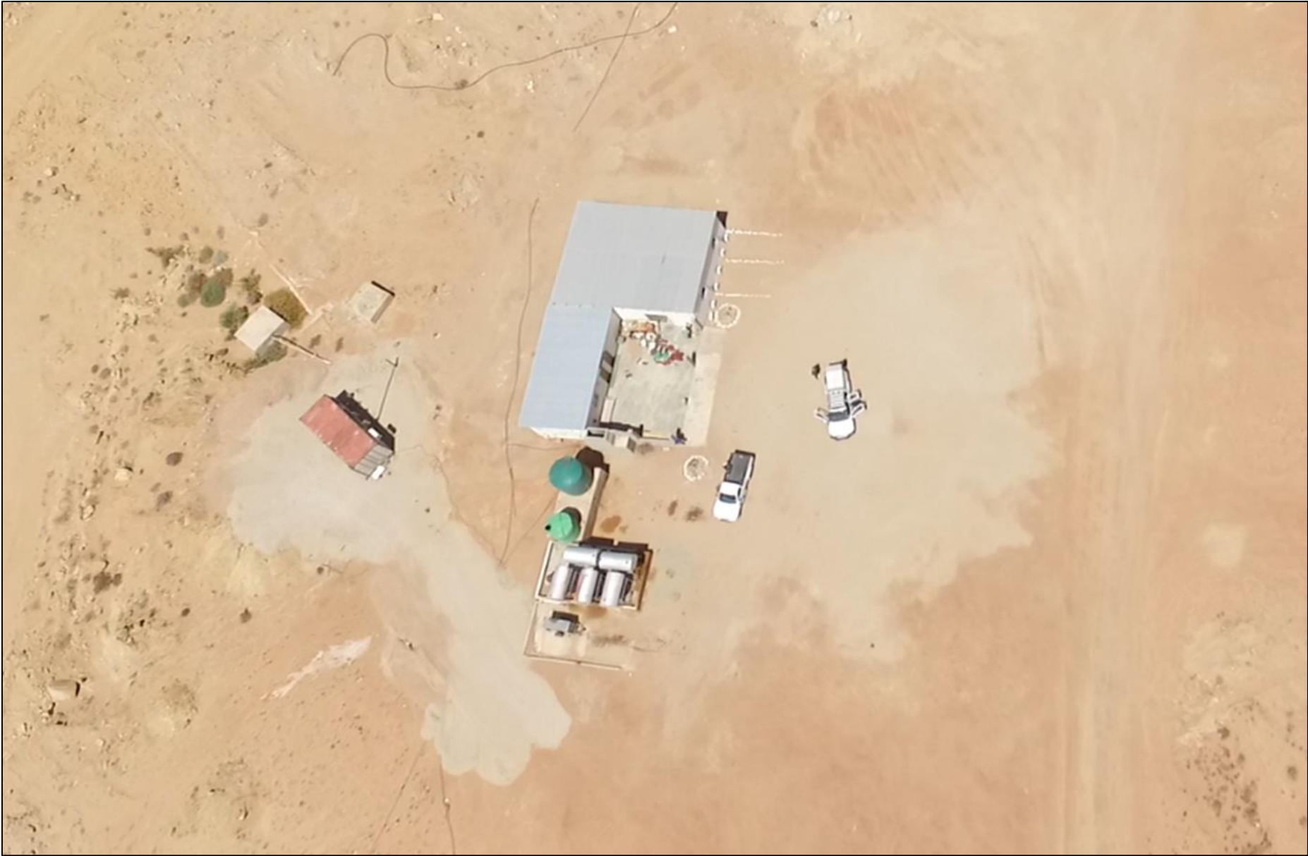
Figure 8: Site Office and fuel supply
