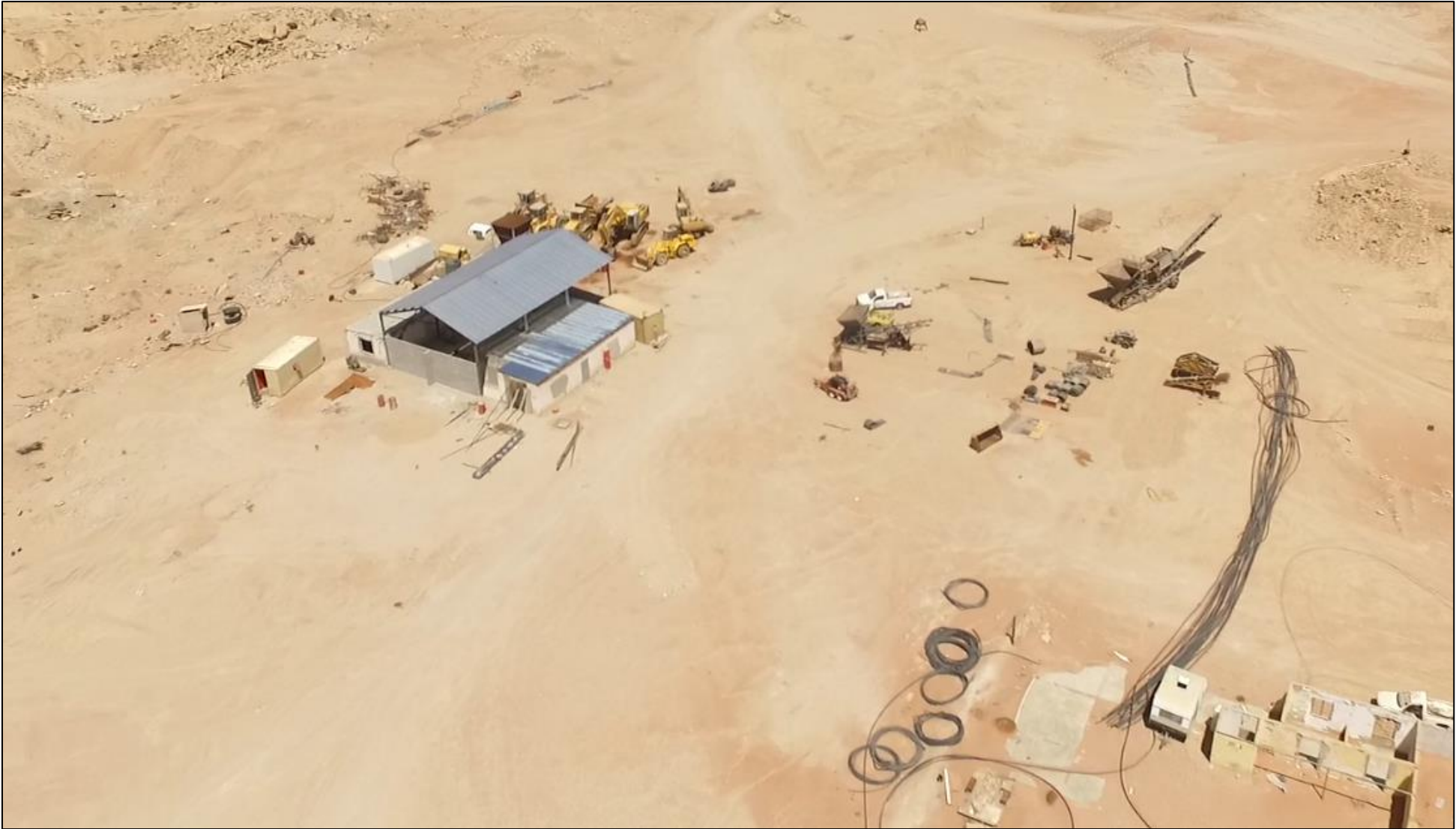
Figure 11: Workshop 2 with parking and laydown area
