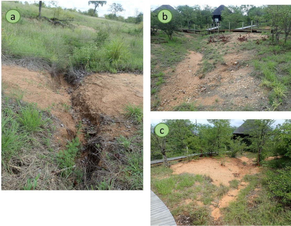
Figure 29: Current route to the drainage line crossing.
