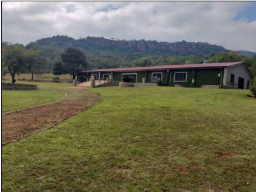
Fig. 4. Site RS 3. The building was built between 2012 and 2013 as evidenced by aerial photos (see figures 4.6 & 4.7). It is a functions venue.
