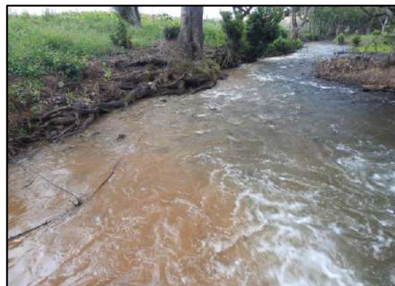
b) Suspended sediments mobilised by equipment washing upslope of culvert over Houtbosloop near TR04. [MU17d, 2018-05-28].
