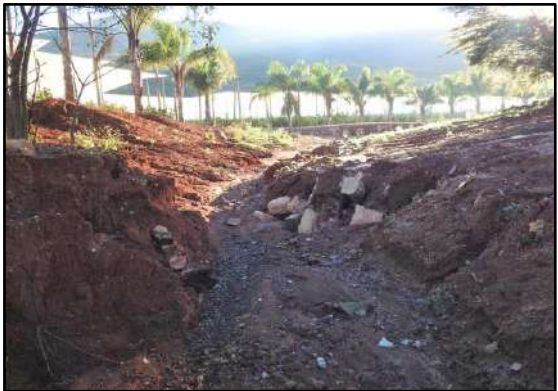
f) Episodic Drainage Line on Koedoeshoek.
