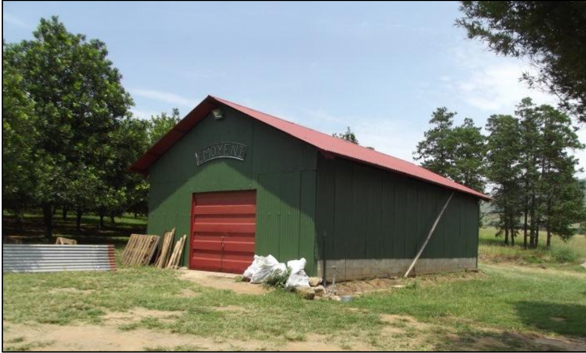
Fig. 3. Site BA 3. A corrugated iron workshop and storage shed.
