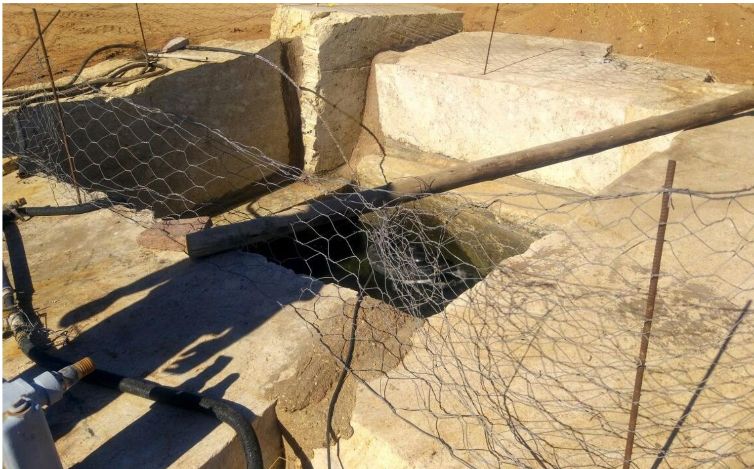
Dam D1 Balancing Dam for Yellow pumps
