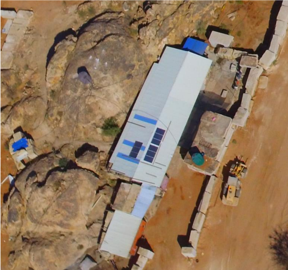
Tanks at Yellow LQ T1
