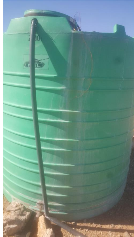
Tanks at Farm Pump T2
