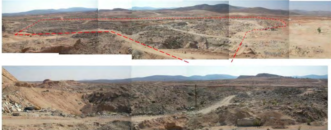
Figure 31: Panoramic view of excavation 4 and overburden dumps 3 to be profiled by means of dozing
