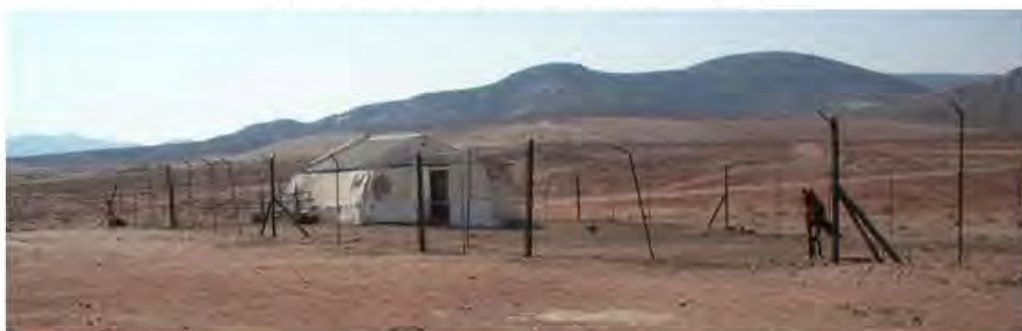
Figure 6: Explosives magazine to be recommissioned or demolished
