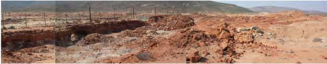
Figure 22: Target 6b to be backfilled and profiled by means of dozing
