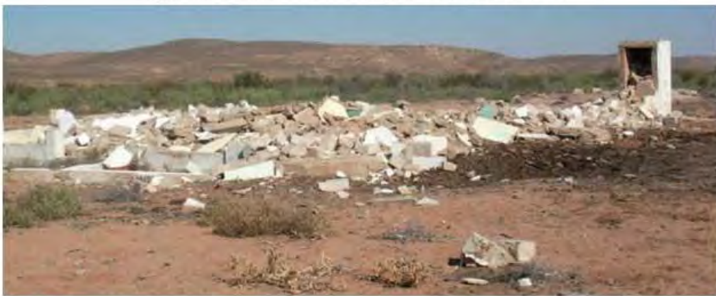
Figure 8: Building rubble to be removed
