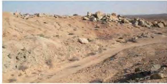
Figure 23: Excavation to be backfilled by means of dozing
