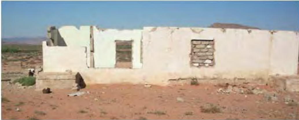
Figure 7: Old farmstead to be demolished and rubble removed
