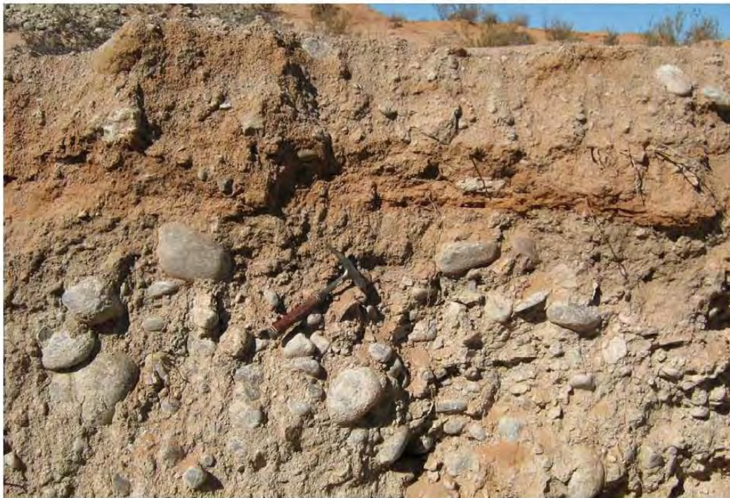
Figure 16: Bulldozed trench Target 3 during mining operations
