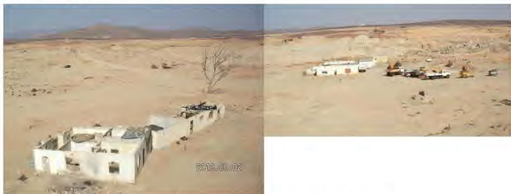
Figure 5: Ruins to be recommissioned or demolished
