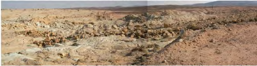
Figure 24: Overburden dumps to be backfilled by means of dozing into existing excavation
