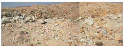
Figure 36: Surface disturbance to be levelled and profiled
