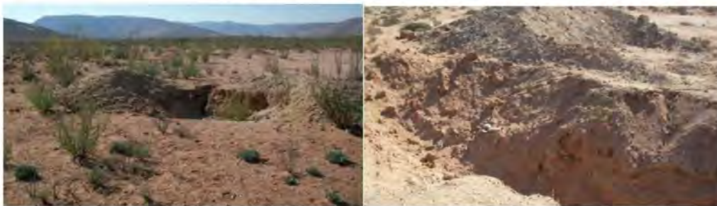
Figure 18: Excavation to be backfilled and profiled
