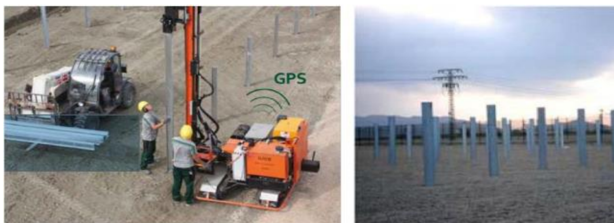
Figure 25: Typical Rammed Piles
