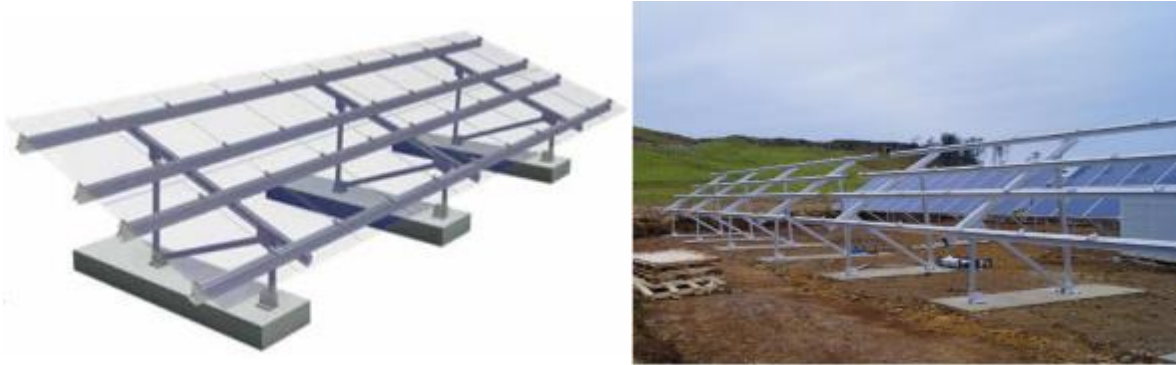
Figure 27: Typical Ballast Foundation
