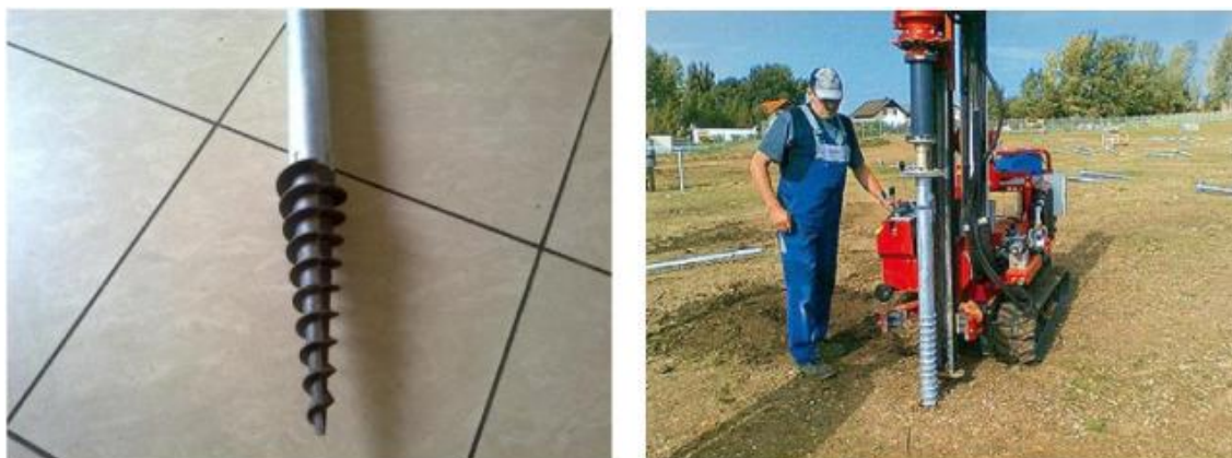
Figure 24: Typical ground screw pile
