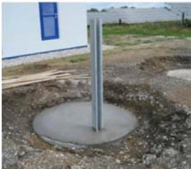
Figure 26: Typical concrete pile foundation
