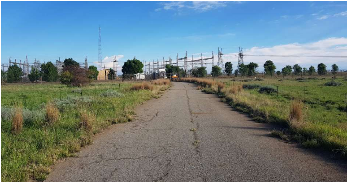
Figure 2: Existing Eskom substation as viewed from the R76 looking north.
