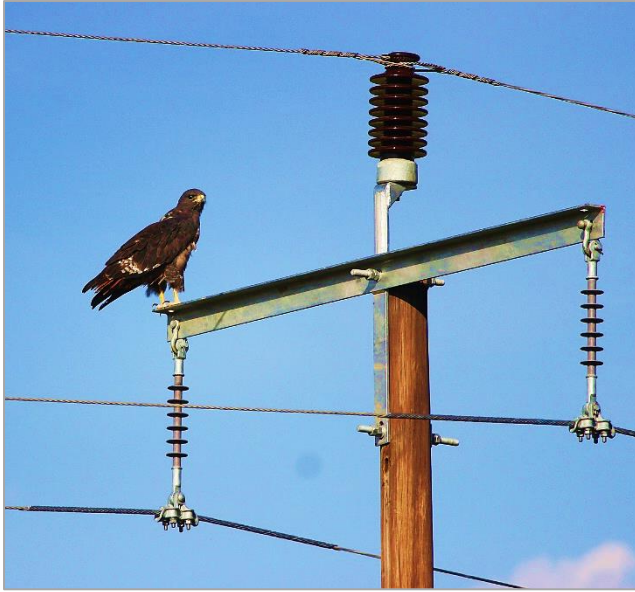
Photo 3a,b,c,d: Making power lines safe for birds of prey, and other species.
