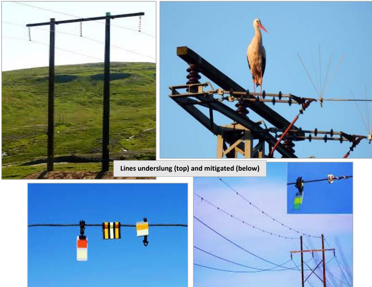
Photo 3a-d (above): Methods used to reduce avian collision fatalities on power lines (by using dynamic bird flappers) and bird-friendly structures (conductors slung beneath the towers) to avoid electrocutions.
