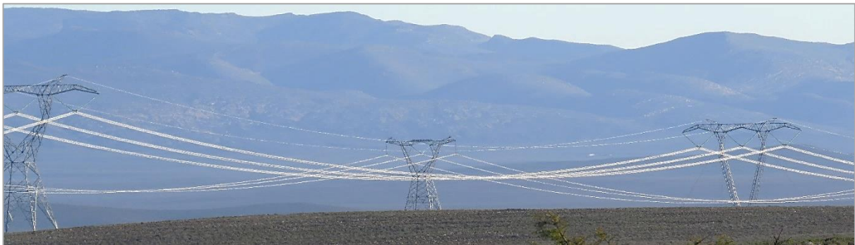
Photo 1: Example of staggered pylons, in which the tower of one OHPL is aligned with the mid-span of the adjacent OHPL in the Karoo. Theoretically, this should decrease the collision frequency of species such as bustards by 67%.
