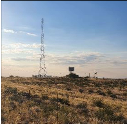
Figure 4: Municipal water reservoir and existing Telecommunications Tower, located approximately 700 m north-east of the proposed PV Block and BESS site, adjacent to Rietfontein town.
