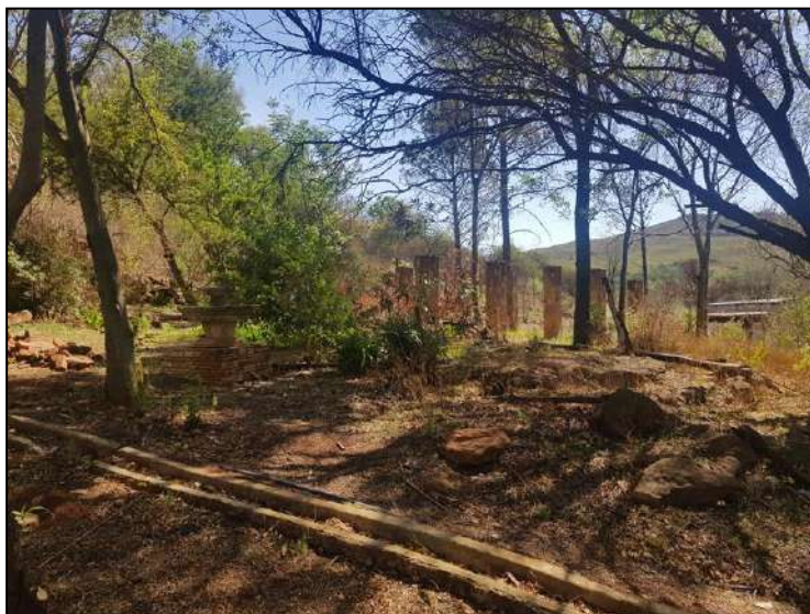
Figure 3-15: The partially collapsed remains of a water fountain (left) and a concrete hedge at the modern residence.
