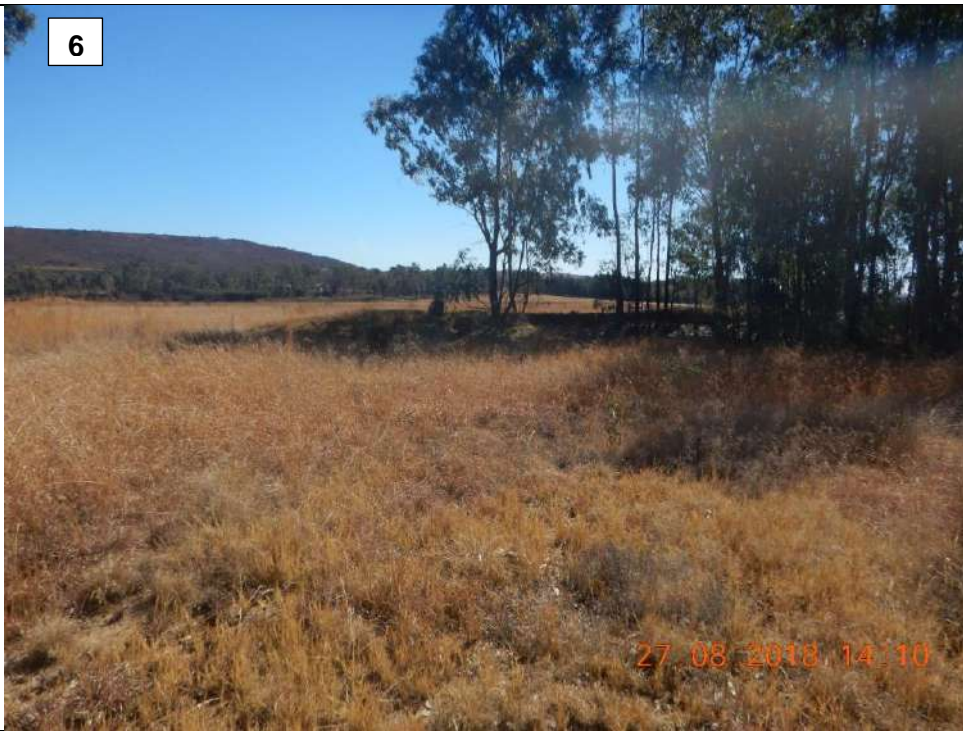
North western view of the small earth dam wall. Co-ordinates: 26°22'49.31"S; 27°57'57.95"E
