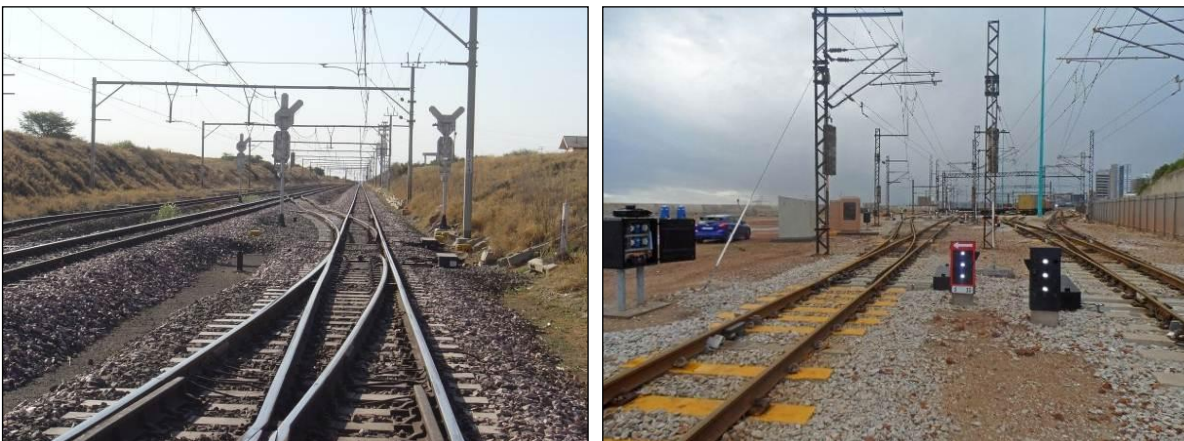
Figure 3.4: An example of a railway perway (left) and typical railway signalling (right).
