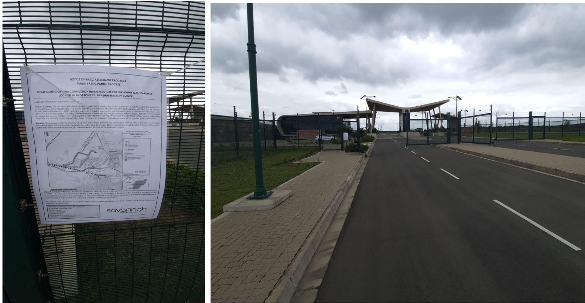
Figure 1: Site notice 1 placed at the entrance to RBIDZ Phase 1F Estate, along Alumina Allee St, Kwa-Zulu Natal (28°44'34.6"S 32°01'59.0"E)
