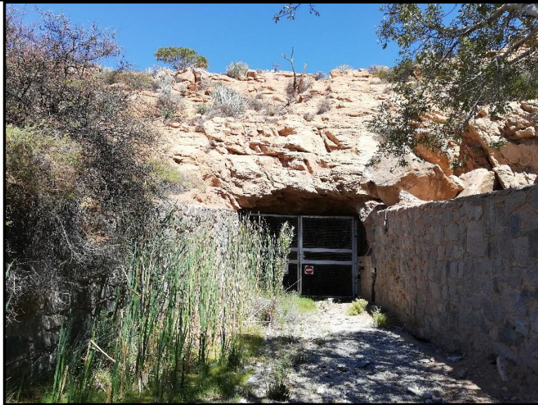
Photograph 6 (dated 30/10/2019): View east of the existing Rietberg Mine Shaft secured to prevent illegal access, where the groundwater is seeping out the mine due to the historical mining activities.
