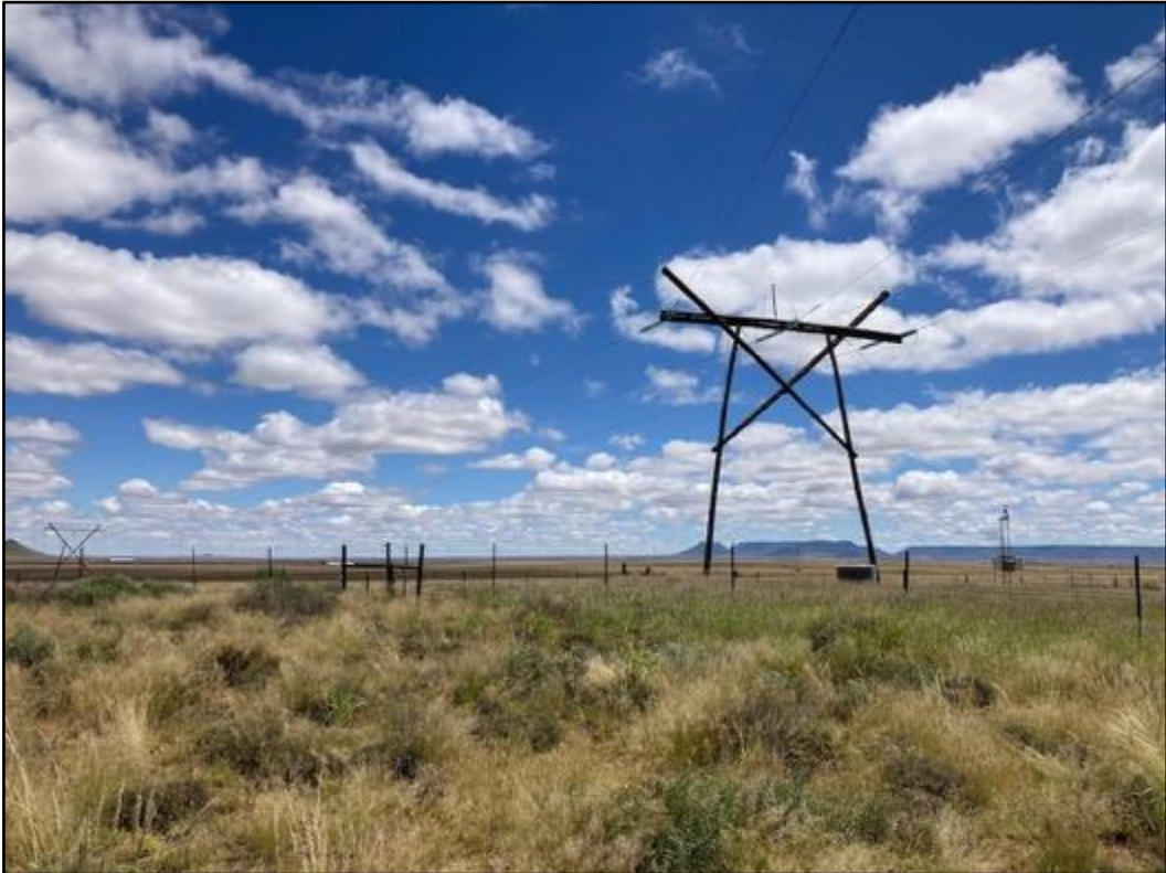
Figure 7: North-western end of corridor.
