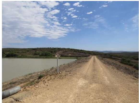
Figure 7: Existing Scheepersvlakte Dam
