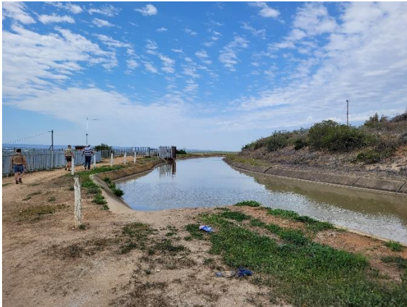
Figure 8: Kirkwood Primary Canal, the source of water for the dam
