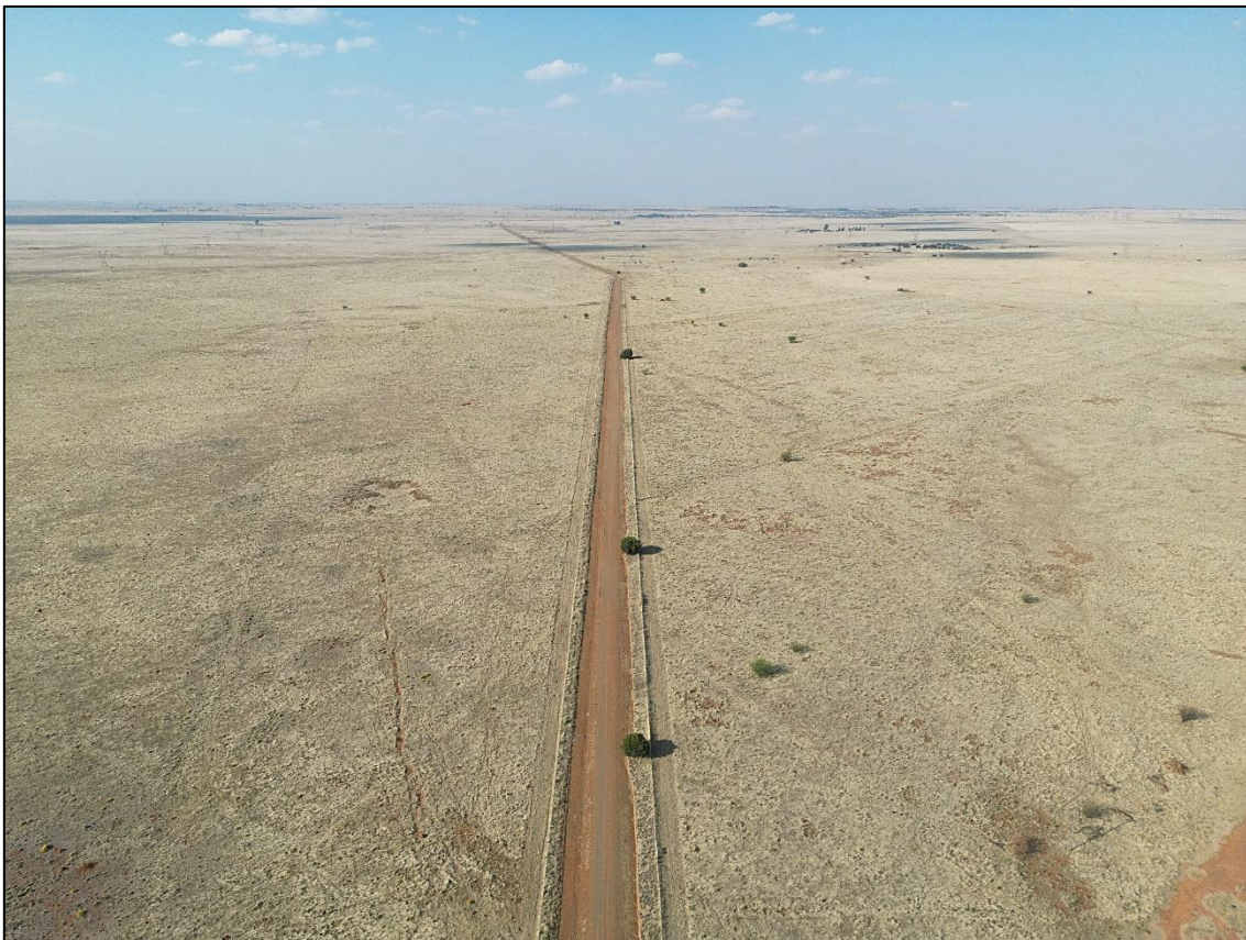
Figure 3.19: 100m AGL area: Taken towards the north-east
