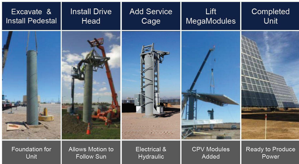
FIGURE 4: ILLUSTRATIONS OF UNIT COMPONENTS AND CONSTRUCTION SEQUENCE
