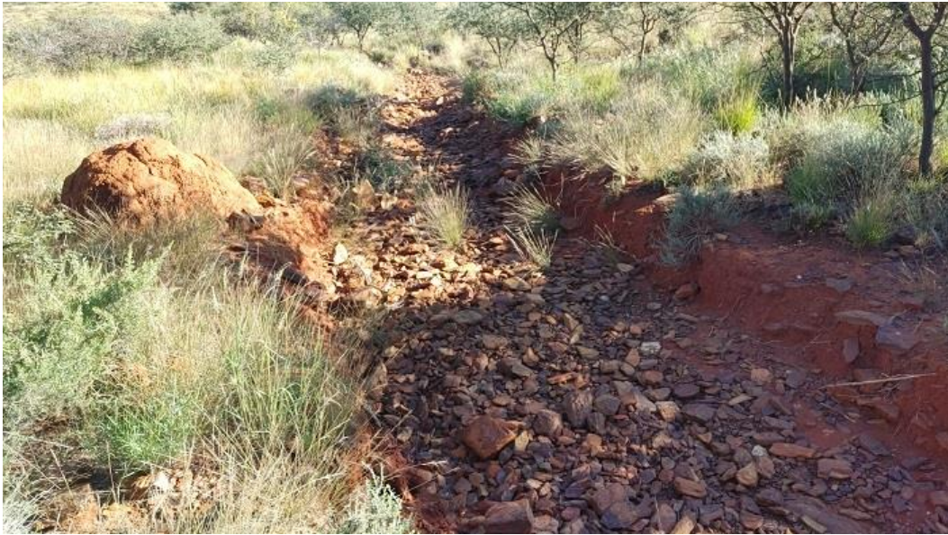
Figure 6: Image illustrating the single significant first-order ephemeral watercourse, which will be traversed by the proposed wind turbine access/service road network and the 33 kV electrical transmission line network with its associated access/service road network, throughout the three mountaintop plateaus
