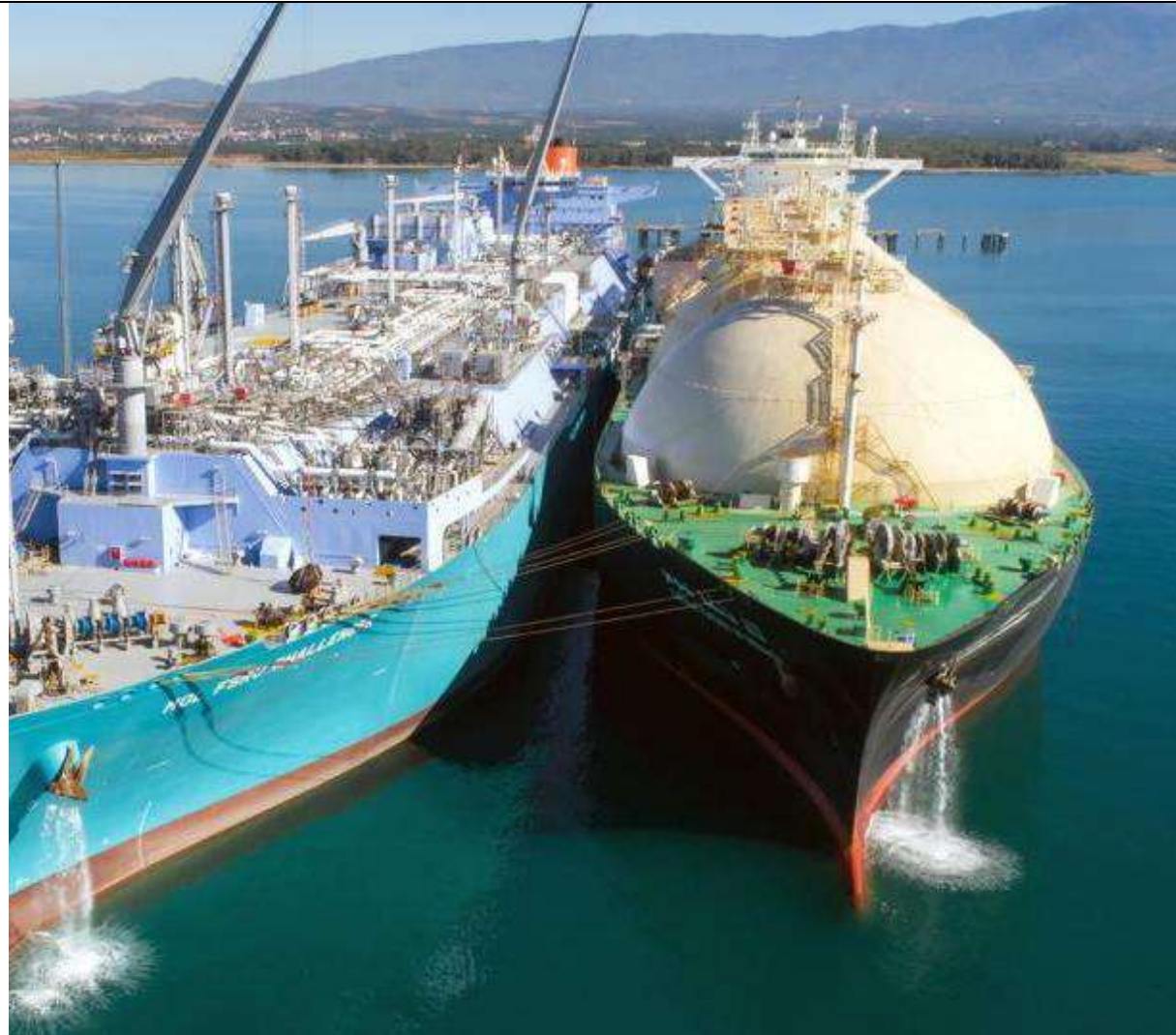
FSRU to LNG Carrier Ship to Ship (STS) mooring for cargo transfer (Source: MOL)
