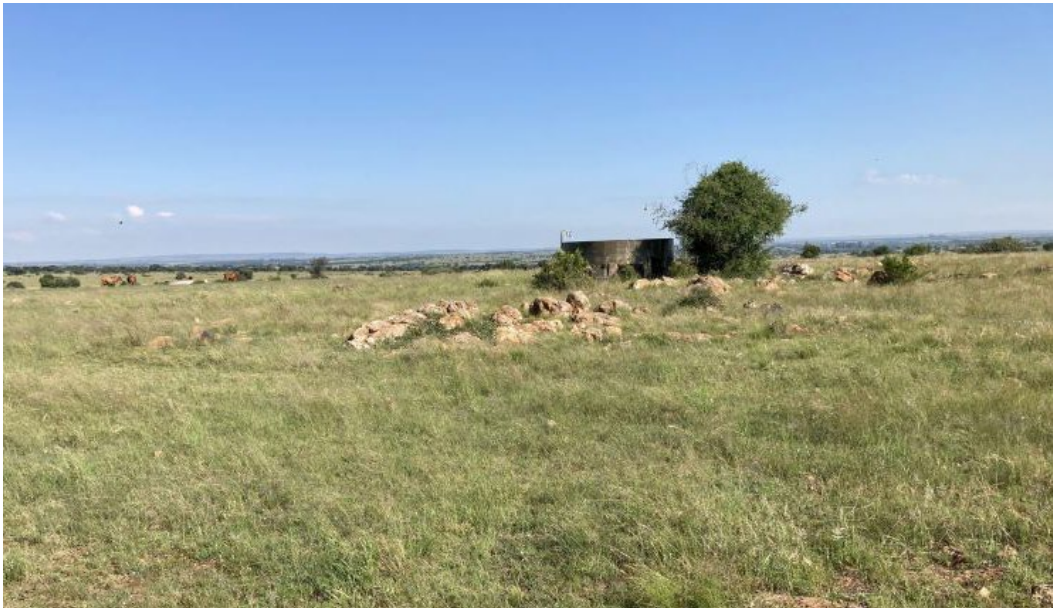
Figure E7: Cement water reservoir in the proposed development area.
