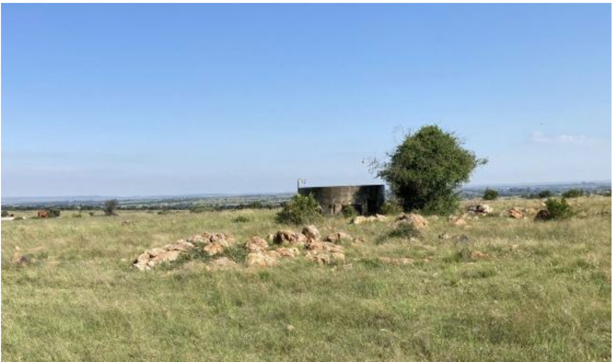
Figure 7: Cement water reservoir in the assessment area.
