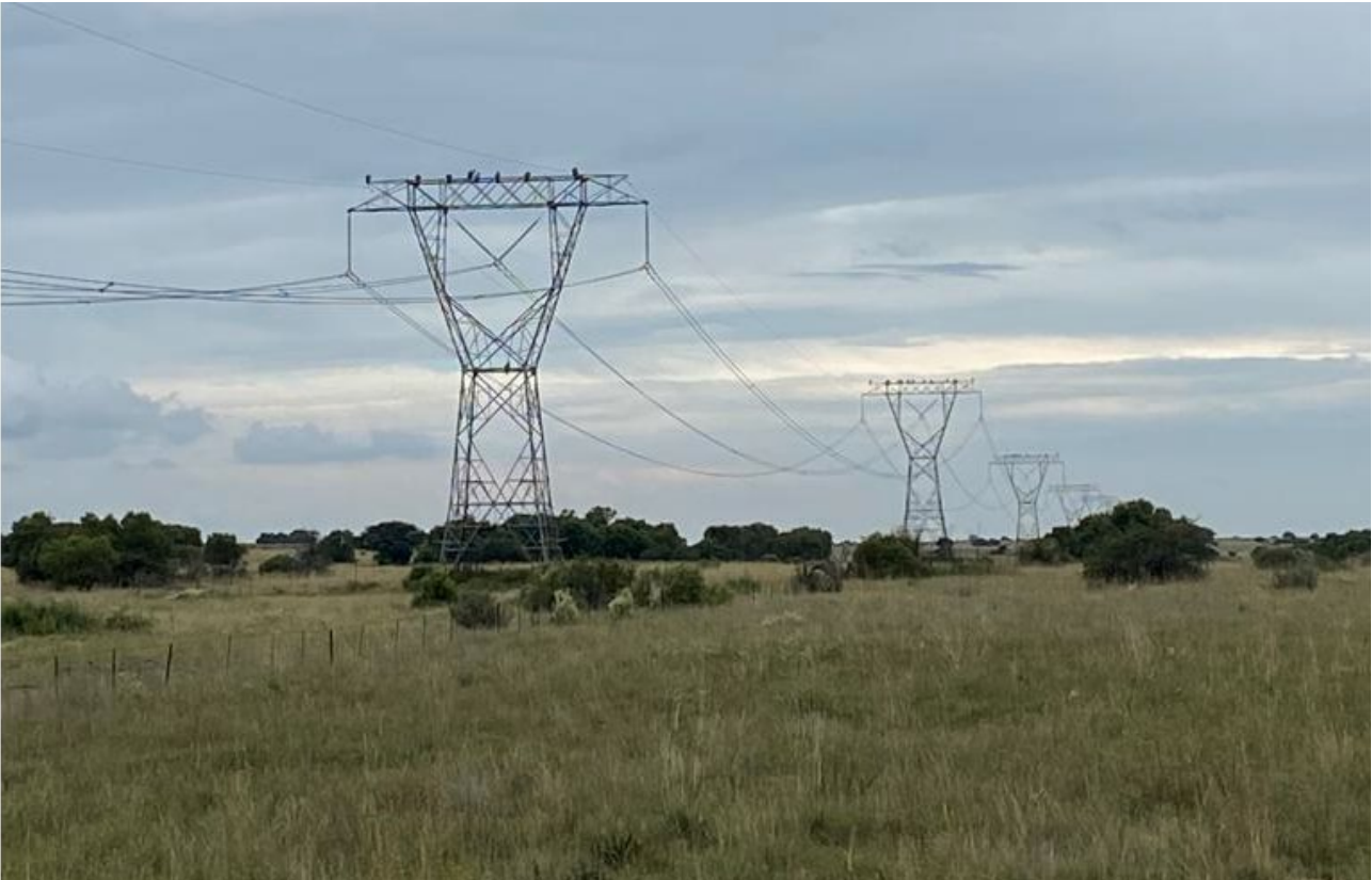
Figure 8: White-backed vultures roosting on the Hermes – Pluto 1 400kV transmission line the assessment area.
