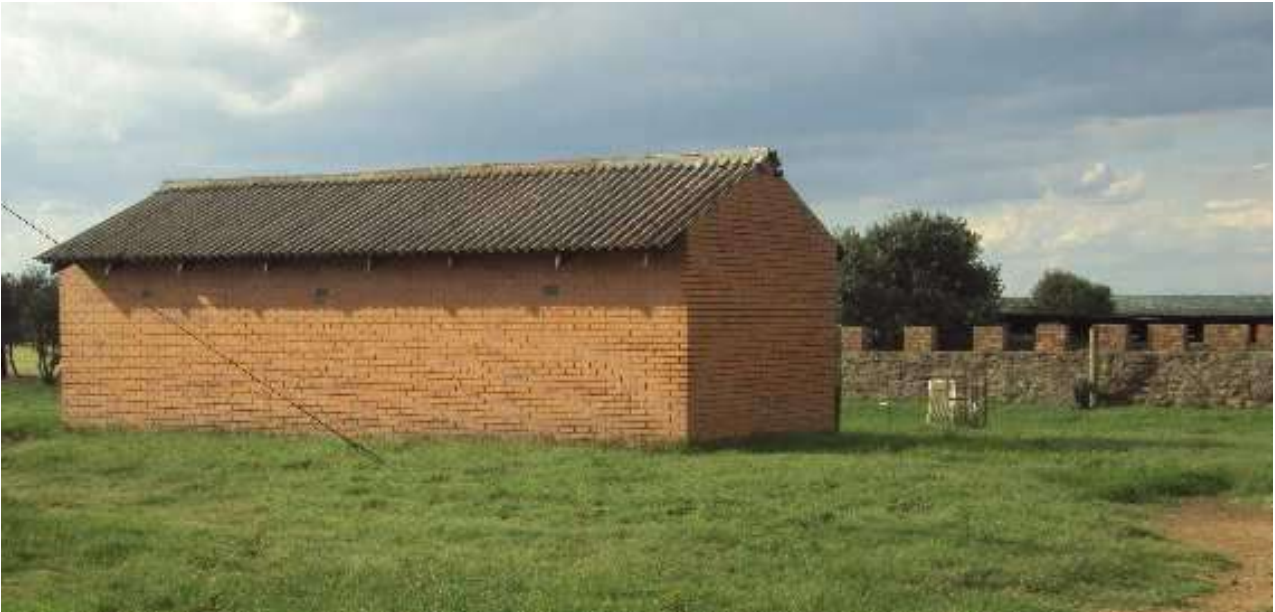
Figure 22: View of the more recent barn/shed, showing part of the historical stone kraal
