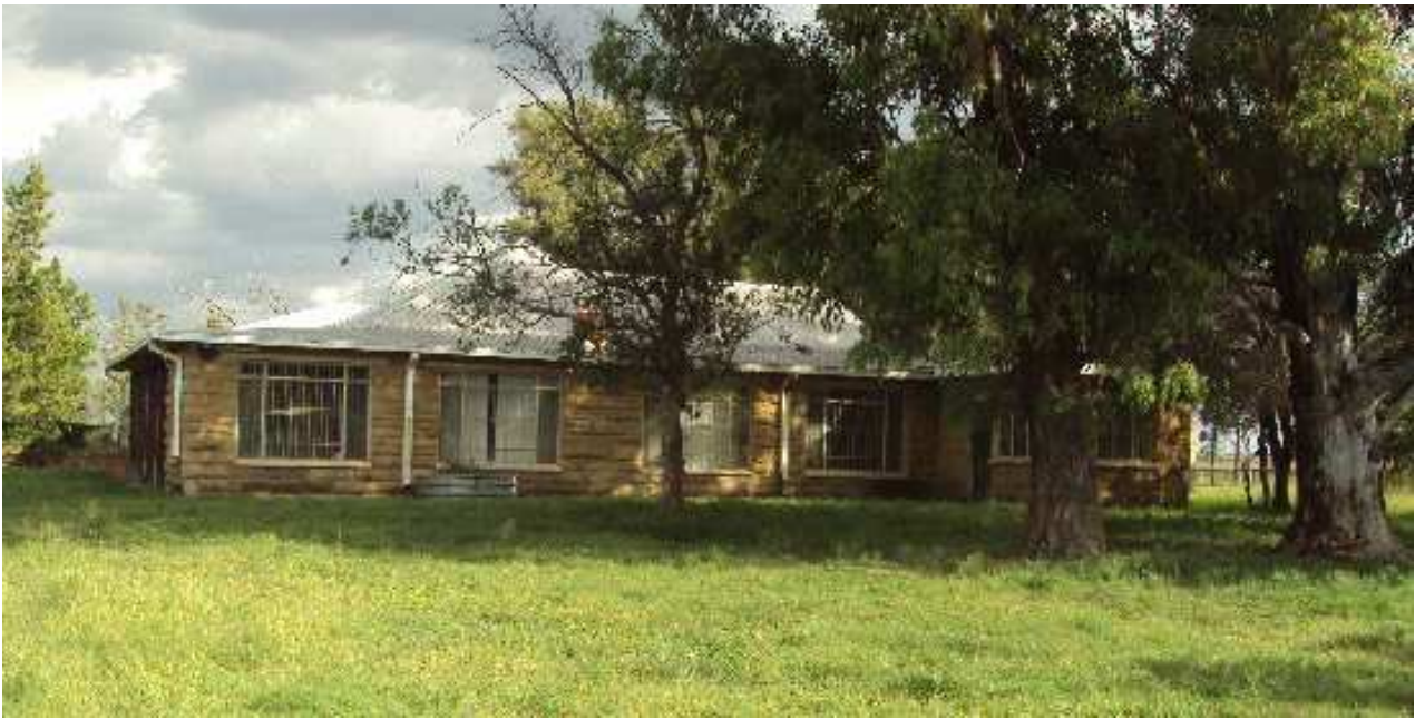
Figure 18: View of the western elevation of the sandstone farmhouse, facing the gravel road
