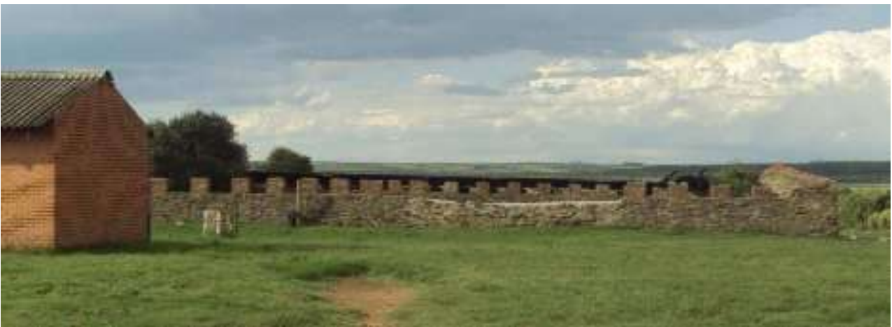
Figure 23: View of the historical kraal, showing brick additions to the stonework
