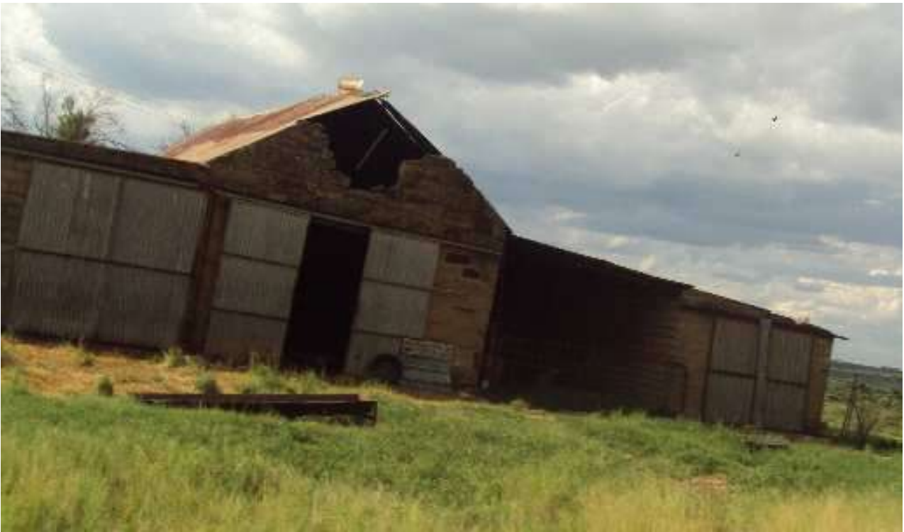
Figure 20: View of historical bar/shed structure, showing later additions
