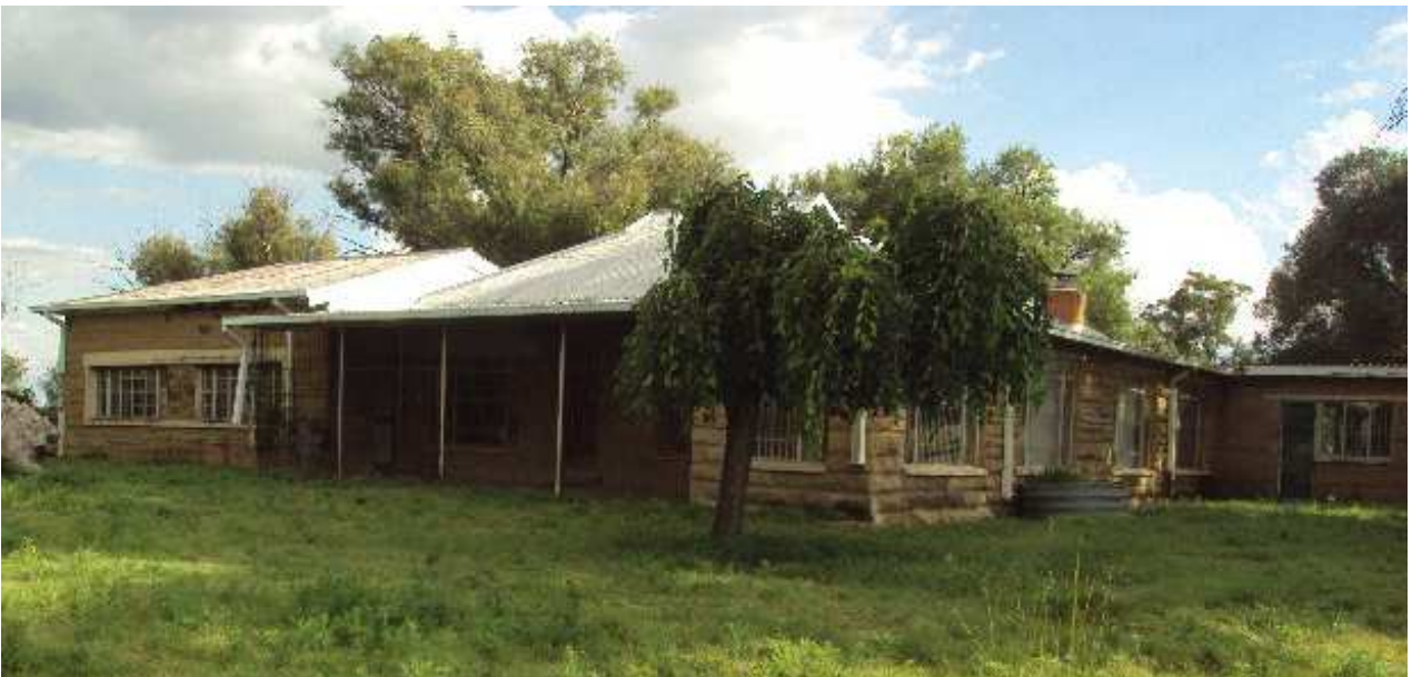
Figure 19: View of the main farmhouse, showing later additions to the original building
