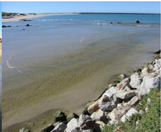
Photo 24. Looking across Coega River Mouth to sandy beach and Eastern Breakwater
