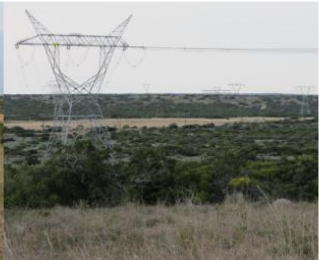
Photo 8. Looking across the Brak River valley to the route of the Rail Link from Bontveld into Thicket and Grassland before joining the existing Railway Line
