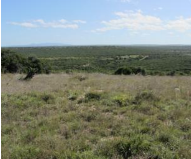
Photo 9. Existing Rail Line in the Brak River valley that will be doubled up. From Dedisa Sub-station
