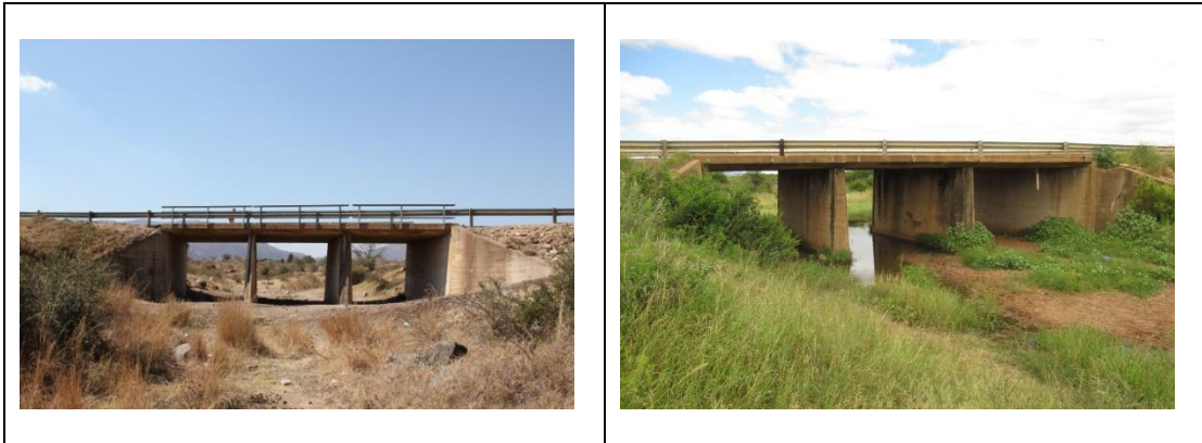
Figure 20. Views of the bridge
