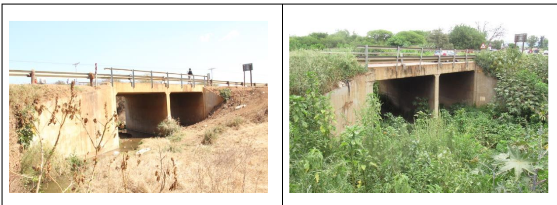
Figure 18. Views of the bridge
