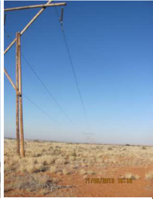
Plate 7: Showing the existing 132 KV power line .
