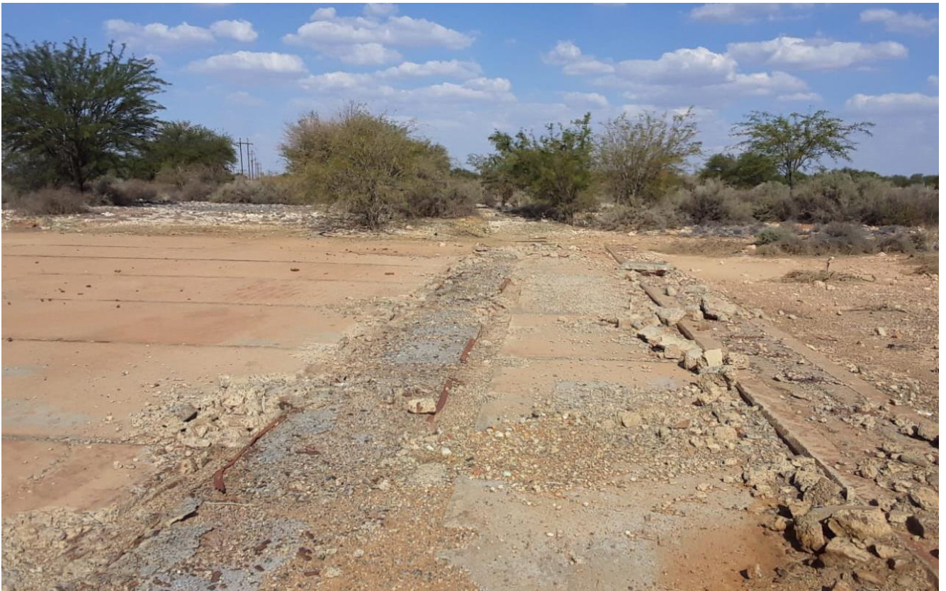
Plate 2: Photo 2: View of old demolished building 20m west of the substation (Photograph © by Author 2021).
