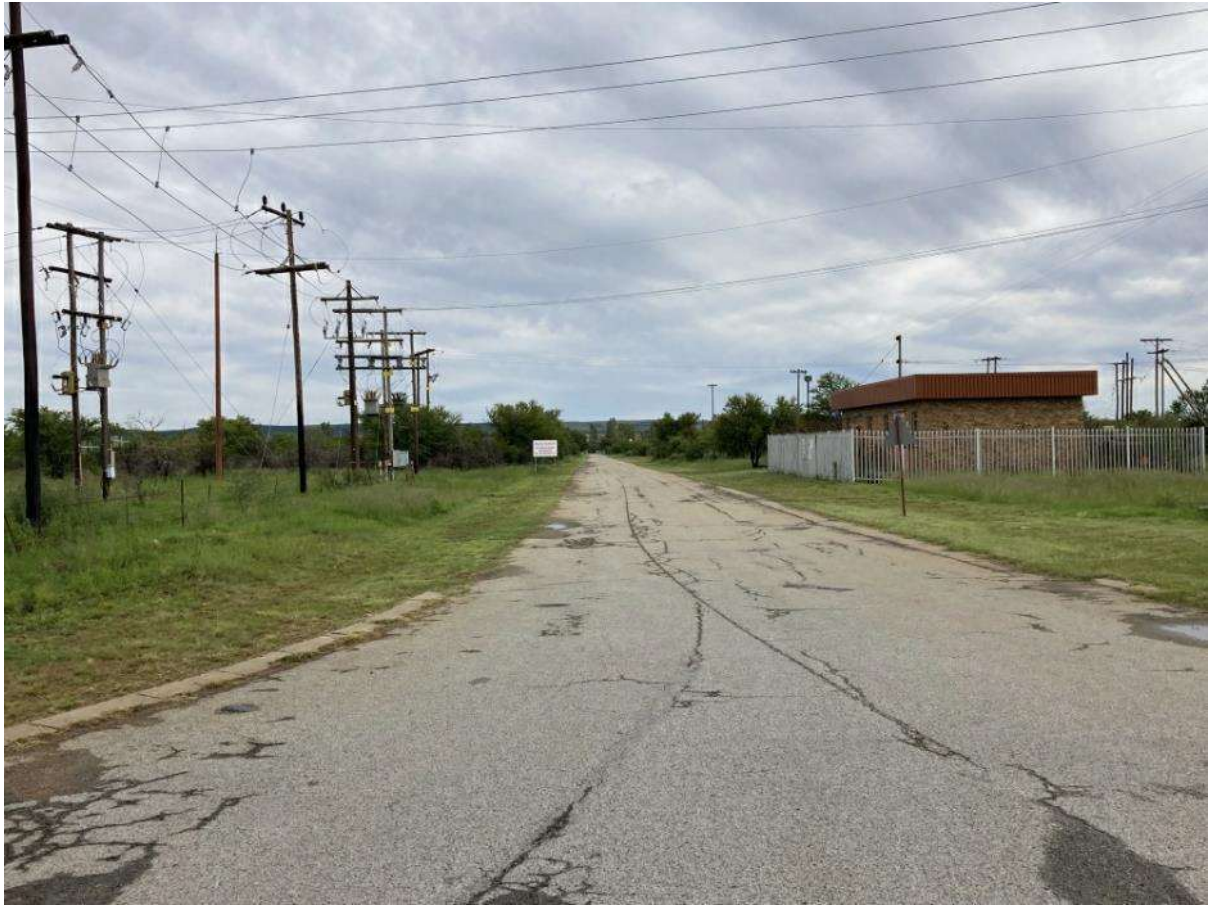
Figure 21: Electrical substation located on the eastern edge of the study area.
