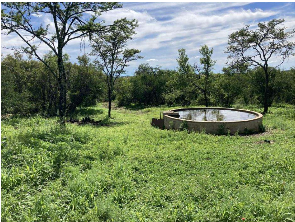
Figure 19: A water reservoir with a cement dam in the study area.
