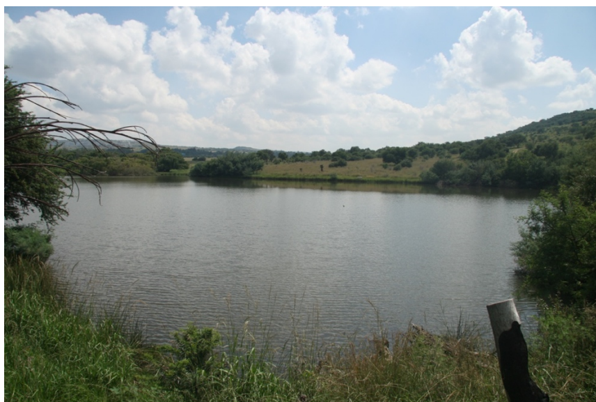
Figure 21. Dam in the Kraalkopspruit.
