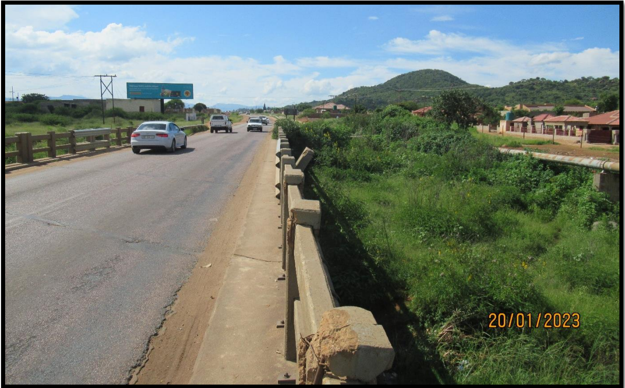
Figure 7: View at second bridge.
