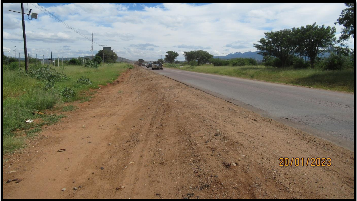
Figure 9: View in south moving towards end of upgrade.
