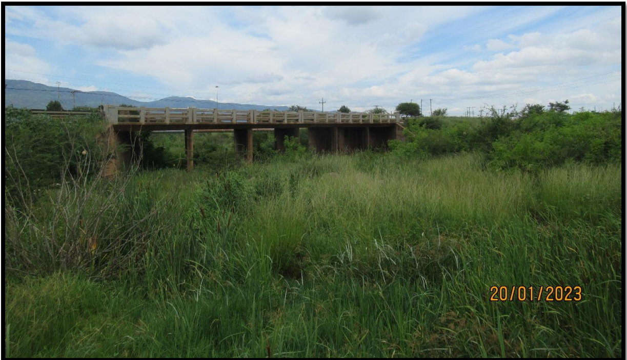
Figure 18: Bridge close to Mokopane.
