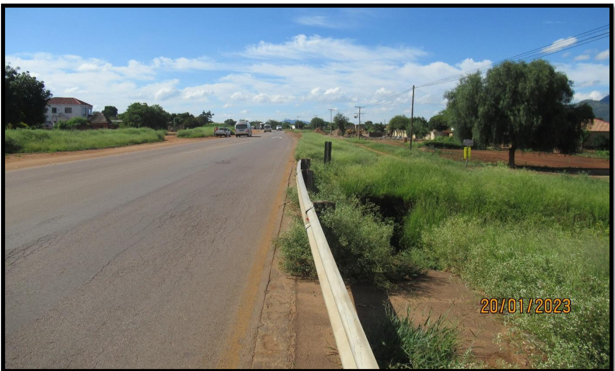
Figure 6: View of road directly outside Mokopane, note bad road surface.
