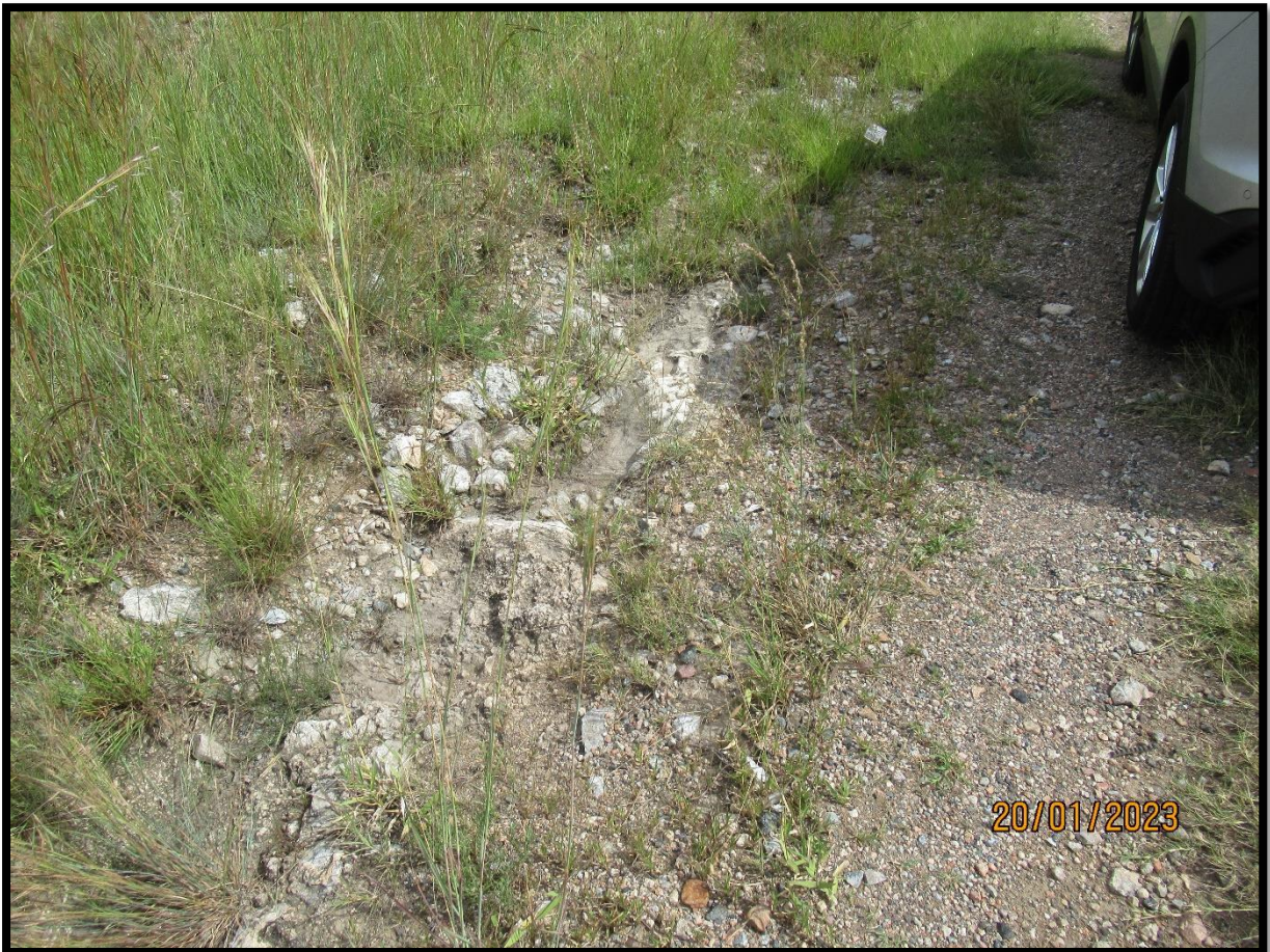
Figure 12: Shallow dolomite outcrop on shoulder of road.
