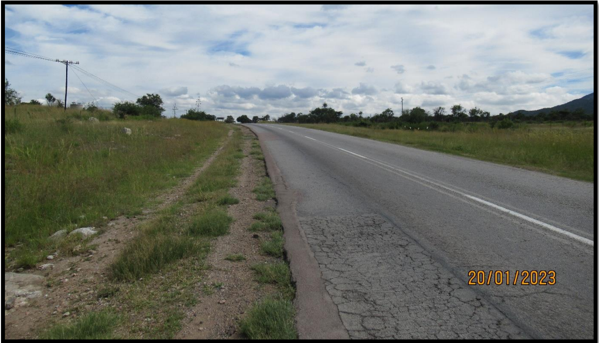
Figure 13: Very bad road surface and shallow dolomite outcrop.
