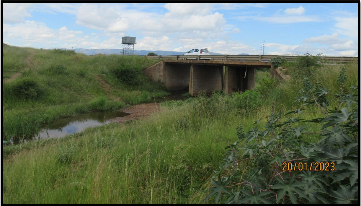
Figure 17: Another bridge to be upgraded.
