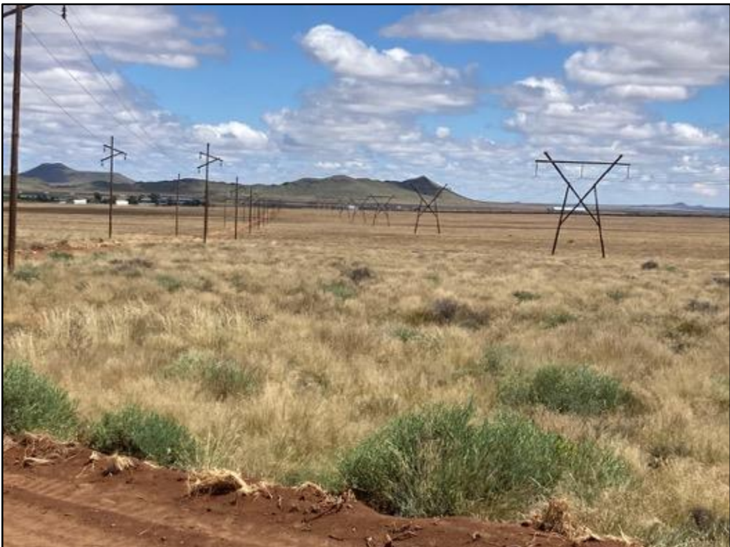
Figure 12: View along existing powerline towards PV2.
