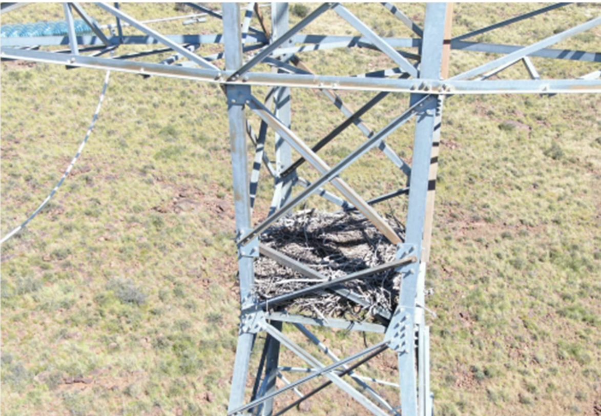
Figure 4: A Verreux's Eagle nest in a high voltage line at the project site.
