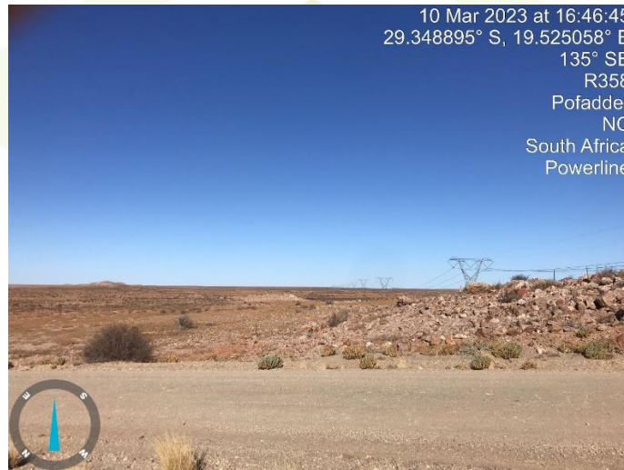
Figure 4.10: Powerline viewed from the R358
