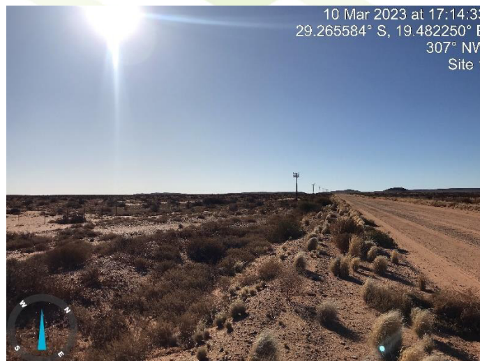
Figure 4.11: Wooden utility poles along the R358
