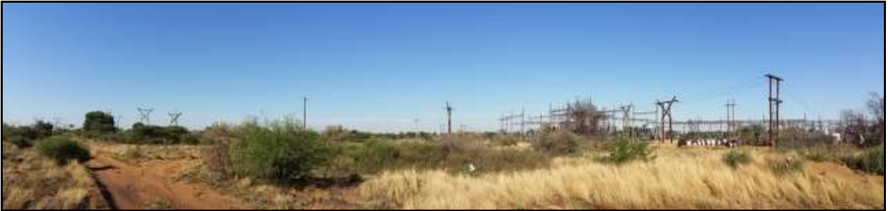
Figure 10: The Hotazel substation on the western edge of the town.
