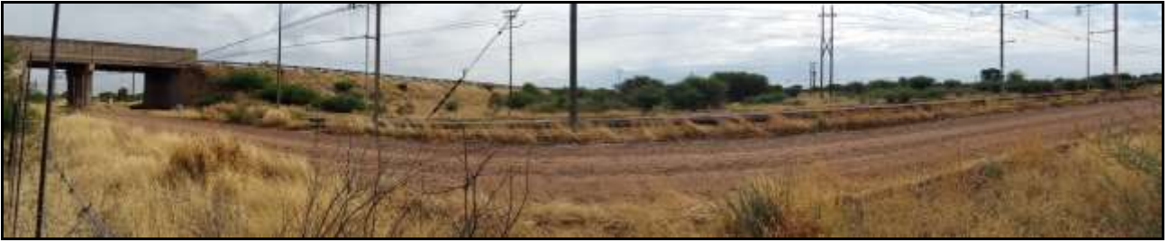
Figure 6: The western half of the Remaining Extent of farm York A 279 has been bisected by the railway line to Hotazel. The R31 crosses the railway line over the bridge shown to the left, and then travels northward, following the railway line.
