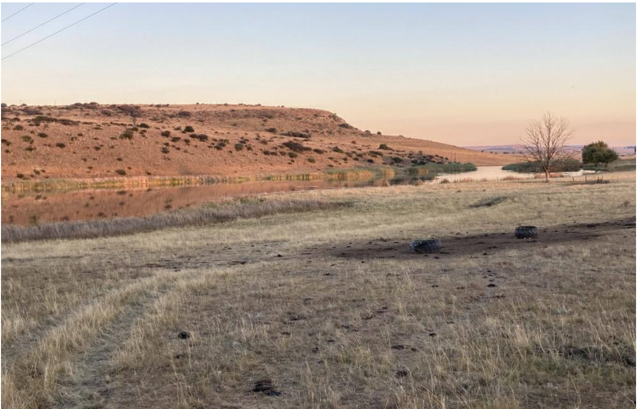
Figure 3: An example of an earth dam in the broader area.
