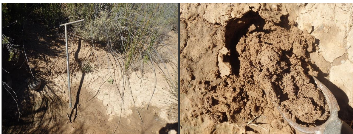
Figure 14: (Left) the embankment of the wetland channel consists of a thick clay layer above impermeable rock. (Right) the soil auger samples consisted of high clay content that was noted to be saturated, however no other hydrogeomorphic indicators were present.
