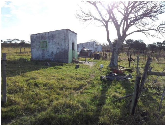
Figure 11: Existing formal houses
