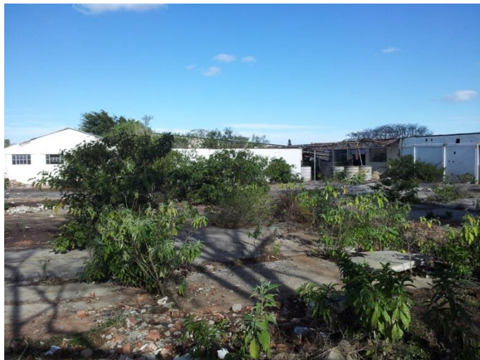
Figure 14: Derelict pineapple processing facility
