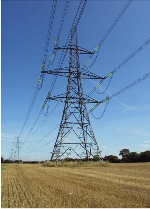
Figure 1: South African examples of the impact HV pylon footprints make on existing biodiversity whether it be cultivated lands/monocultures, or natural veld/grazing. A monopole structure would have proportionally less of an impact on the surrounding environment.
