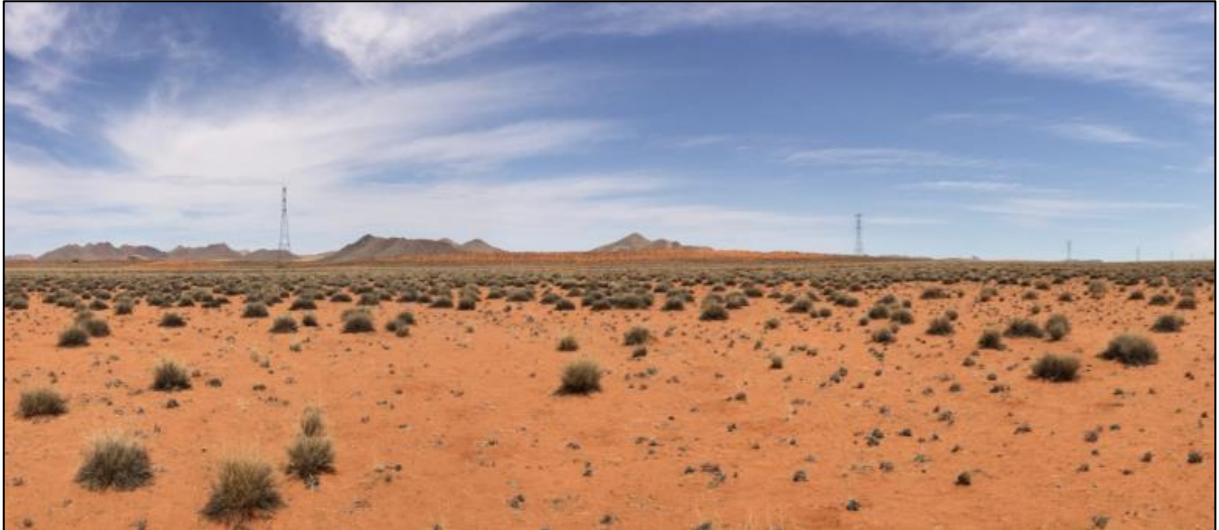
Figure 23: Photograph of the Eskom 220kV power line as seen from the proposed preferred North site.
