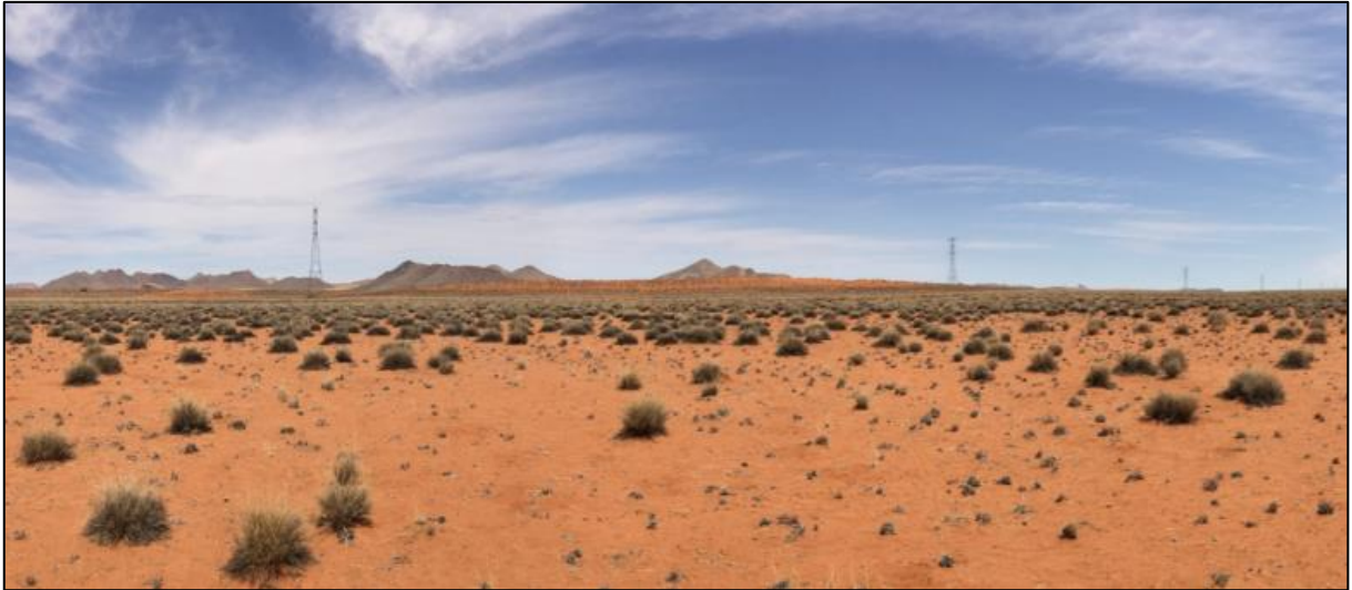
Figure 21: Photograph of the Eskom 220kV power line as seen from the proposed Southern site.
