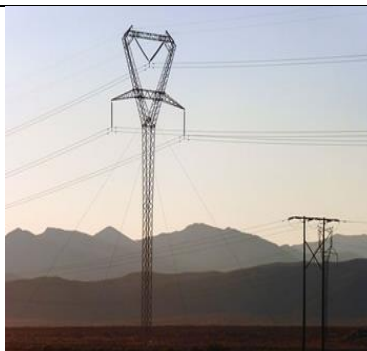
Plate 6-2: Guy line supported steel structures.
