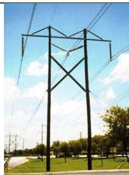
Plate 6-4: Multi-pole structures such as H-towers or K-towers.
