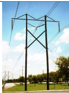
Plate 6-4: Multi-pole structures such as H-towers or K-towers.
